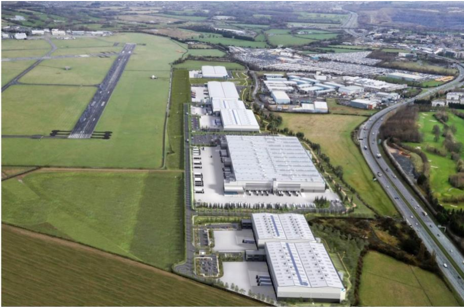
Mountpark Baldonnell scheme is just off the N7 in Dublin 22
